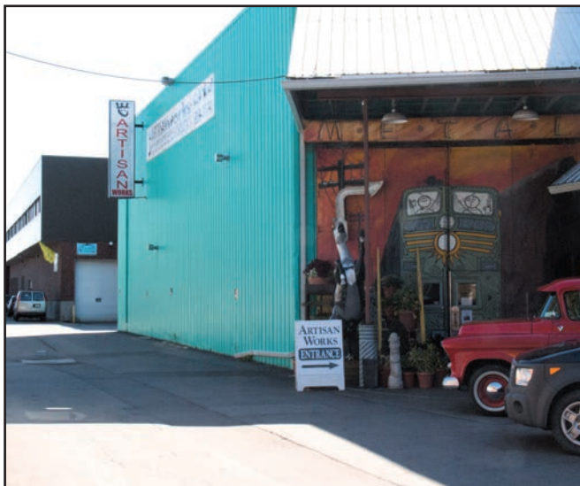
Fig. 1. Situated in a repurposed industrial complex, the entry door to Artisan Works gives a hint that the unexpected can be expected upon entering.
