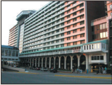
The facility, whether a convention center, religious retreat, or fairground, goes about its daily business as the woodturning symposium approaches.
